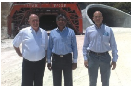
Ambassador at Road No. 6 construction site
